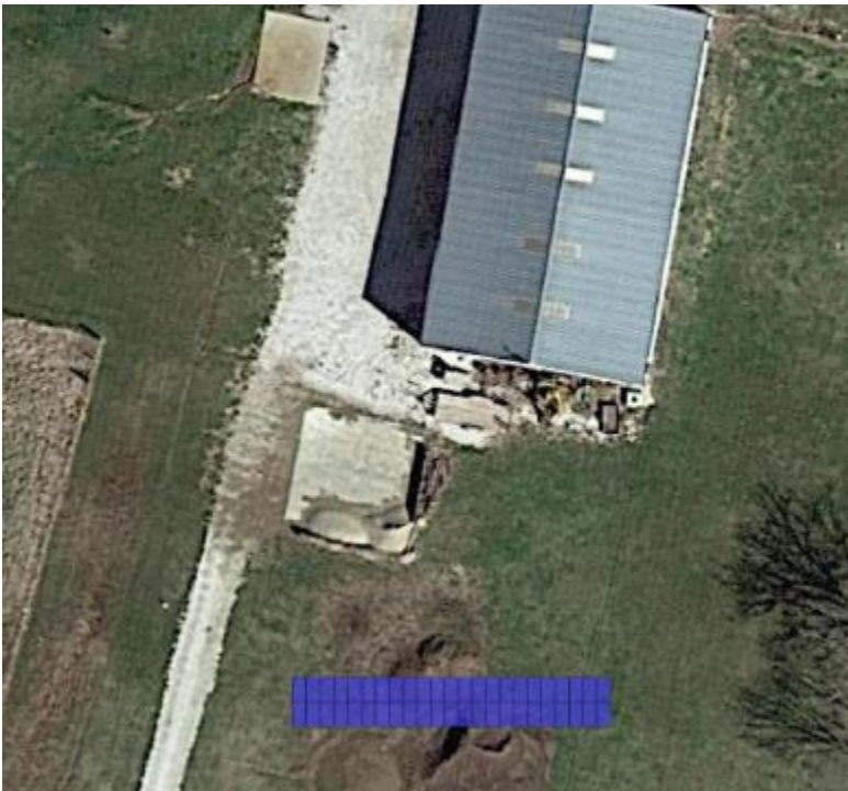
Maintenance: 4092 Hwy JJ
